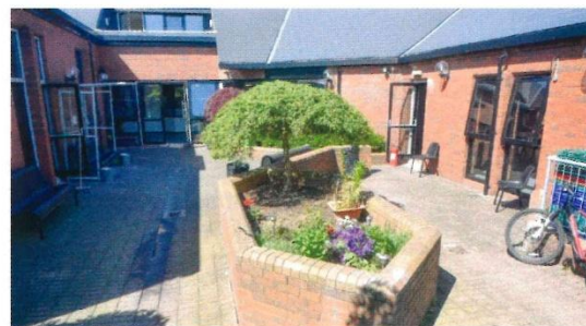
Utility Street Men's Hostel, Belfast
